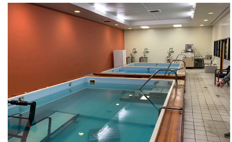
EXISTING RECOVERY POOLS
