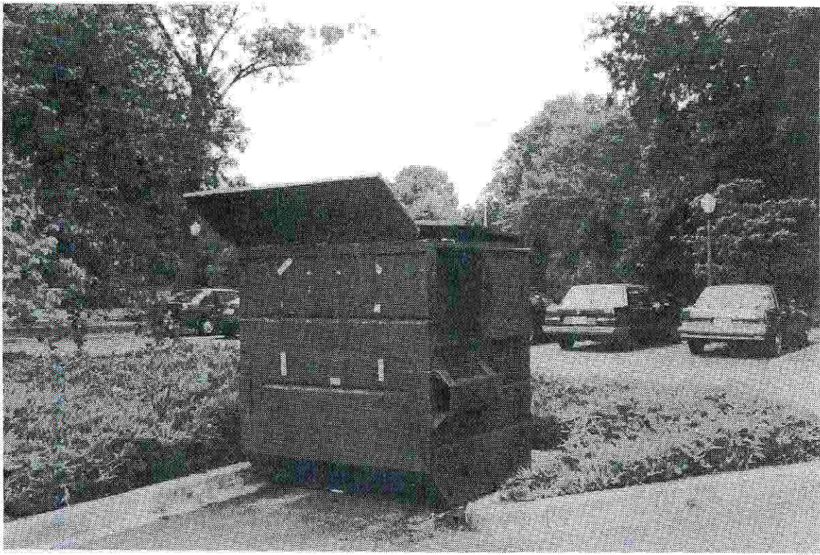
Figure 18: Dumpsters, such as the one in the parking lot behind Sikes Hall, should be relocated or carefully screened by brick walls or landscape materials.
