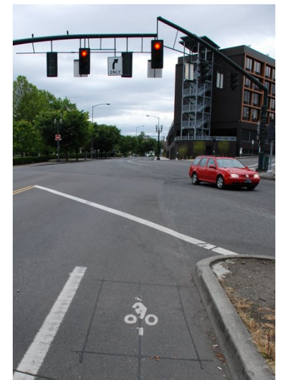
Bicycle-activated loop detector and pavement marking.
