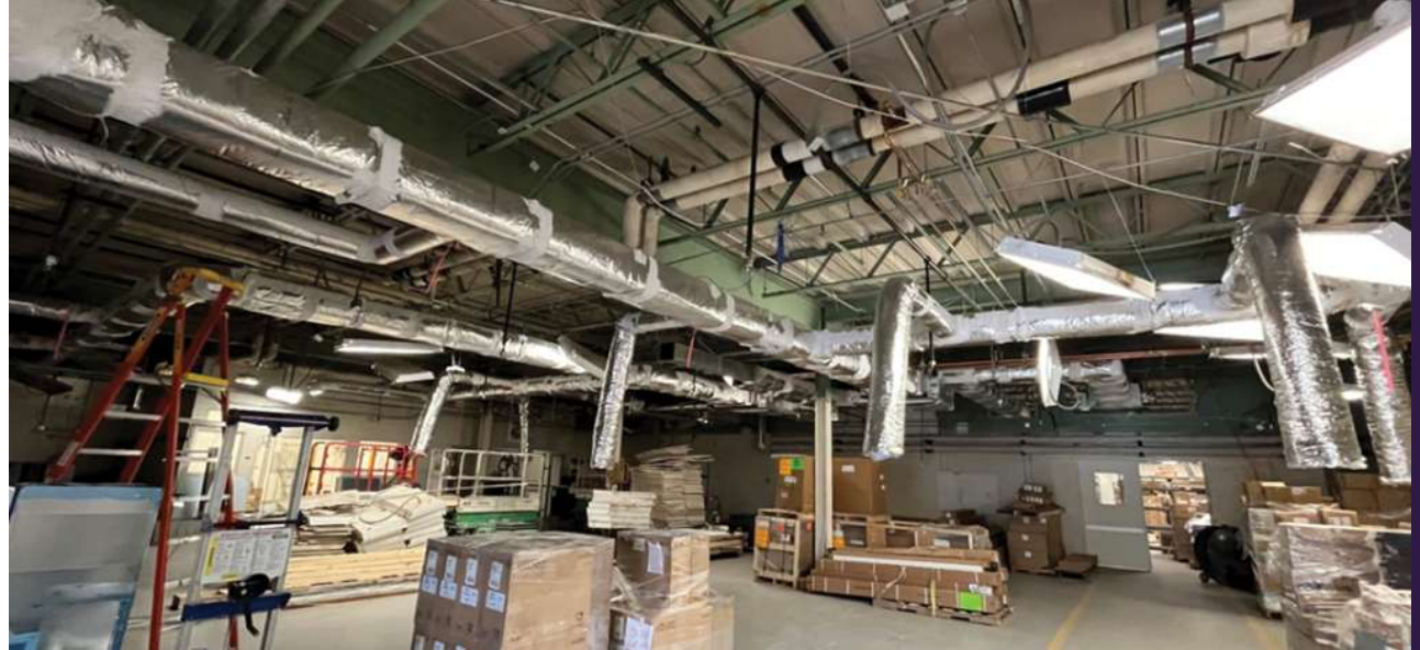
Loading dock storage area of Ravenel where new fan coil units and ductwork are being installed.
